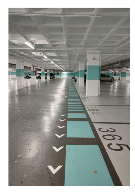
The entire area is painted with polyurethane resin in different colours to create an innovative design that indicates the streets. The same design is applied on walls and columns with special attention to entrances and the reception areas.
